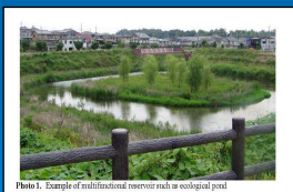
Photo 1. Example of multifunctional retention tank in ecological pond
